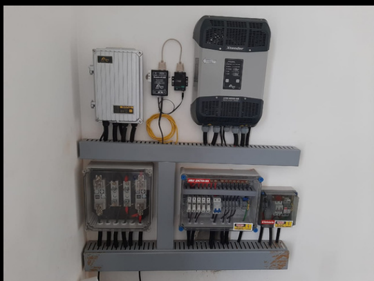
5 KW, STUDER HYBRID, KOZHIKODE
